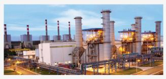
AGP solution. This advanced upgrade technology will expand the efficiency and power output on the site's 9E gas turbine assets. Through this new agreement, GE will install its AGP solution on three 9E gas turbines, which is expected to boost output by 3.4 percent and increase fuel efficiency by 1.7 percent. K-Electric also extended its Contractual Service Agreement (CSA) with GE on the units through 2028.
