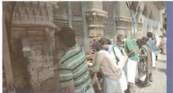
Facade cleaning workshop at Denso Hall
