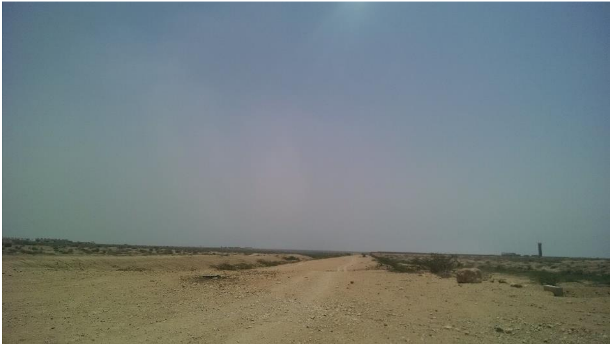
Figure 4.17: ROW of overhead TL in Eastern Industrial Zone, PQA
