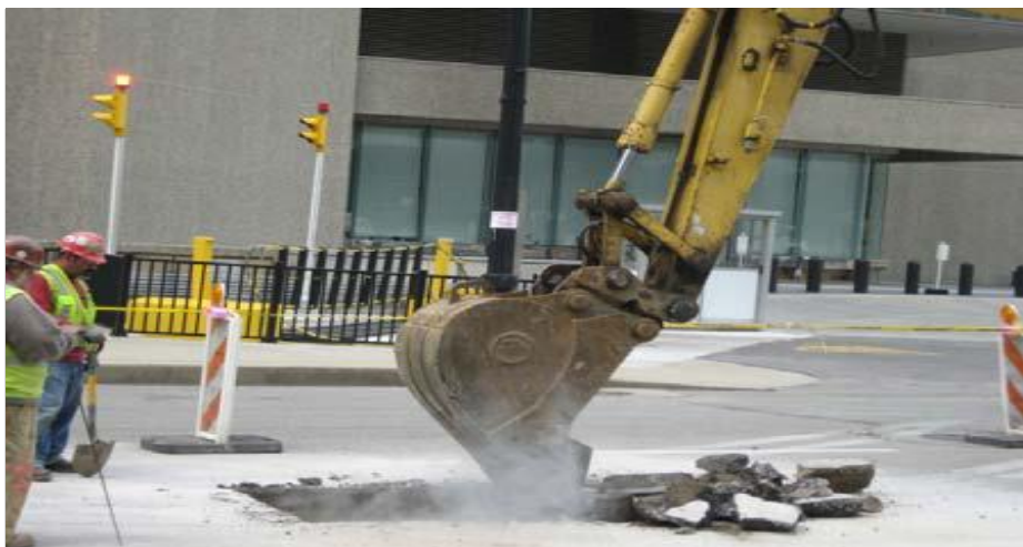
Fig. 2.5: Excavation Using Backhoe
