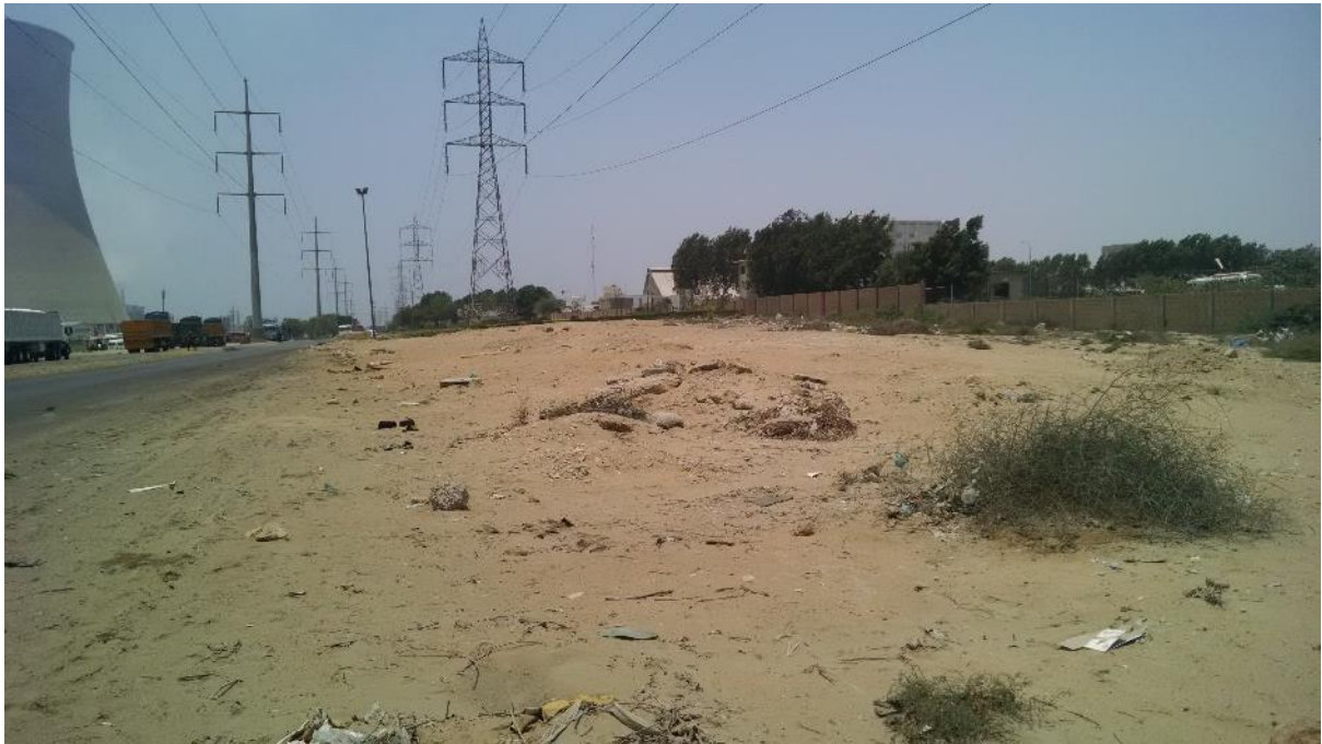
Figure 4.15: Start point of 220 kV TL from Engro Power Plant
