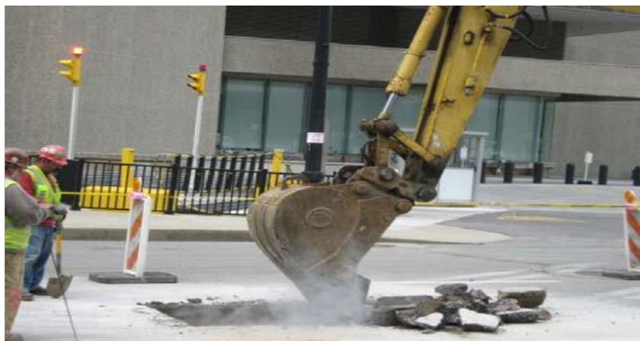
Fig. 2.5: Excavation Using Backhoe
