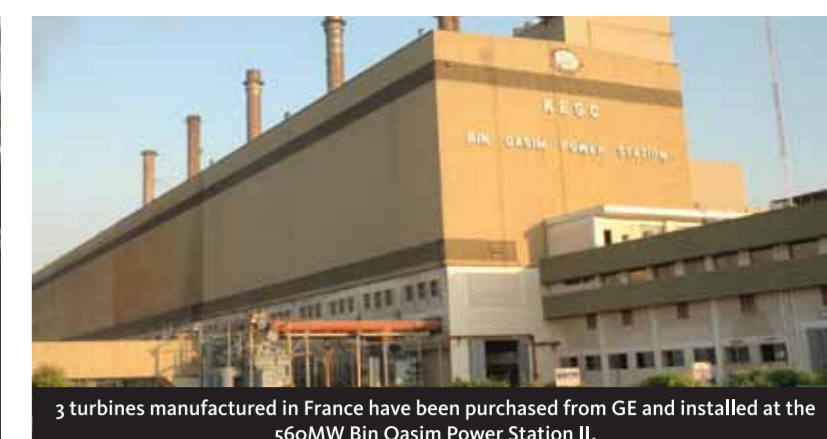
3 turbines manufactured in France have been purchased from GE and installed at the 560MW Bin Qasim Power Station II.
