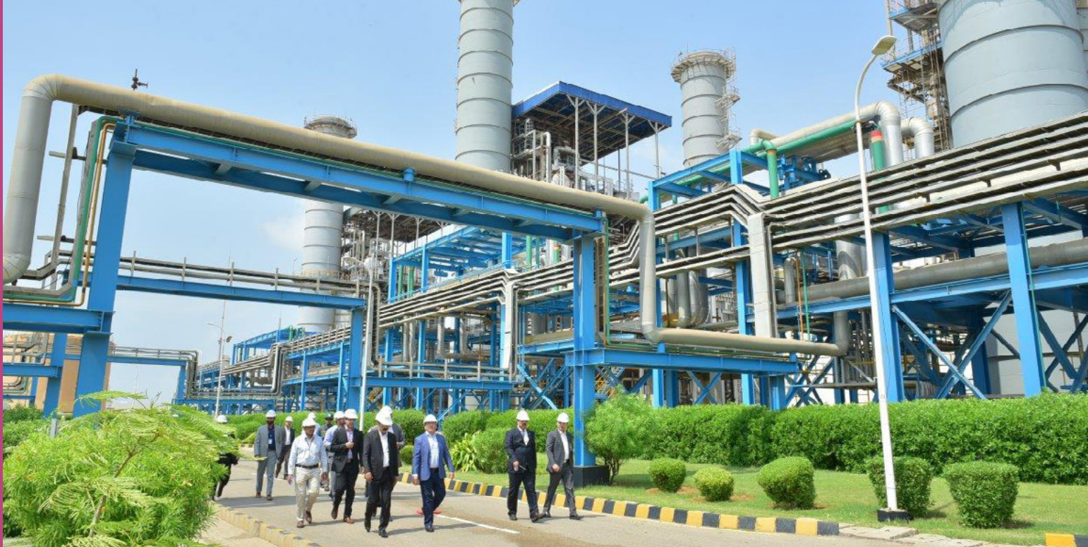
KE Generation Plant - Bin Qasim Power Station (BQPS) II
